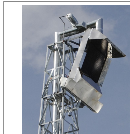
Fig 1. Billboard receiver at the JSS pilot plant [Coventry et al. Solar Energy 122 (2015) 749-762]
